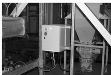
Illustration 1.14: Old solution: Motor control - panel mounted decentrally
