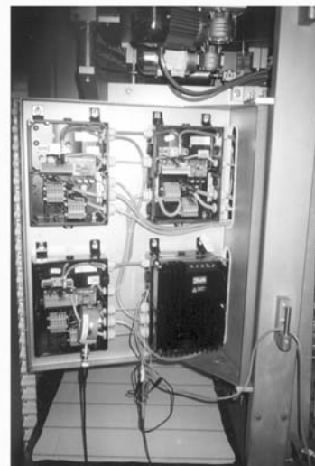
Illustration 1.18: Retrofitting on existing application with speed control
